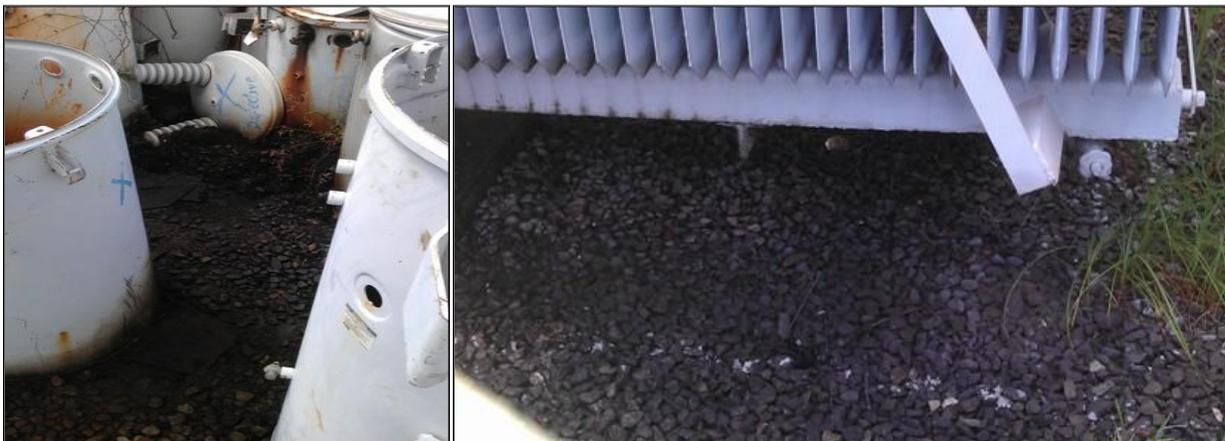
**Figure 2.17 Soil Contamination over 50 ppm associated with stored distribution transformers and an active station transformer - Kingston**
